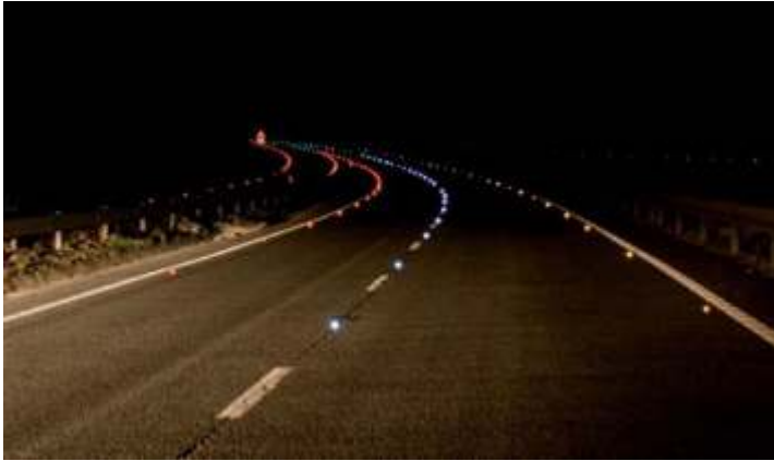
Fig. 2. Intelligent road studs installed in Dover, England [14]
